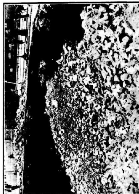
The work of filling up the cavity caused by the landslide at North Quay was commenced yesterday. The lighter Lady Norman operated from the river side, the vessel being shown in the photograph on the left. On land 31 trucks were employed continuously yesterday in dumping spalls into the cavity. The photograph on the right illustrates how far the work has progressed and also gives a view of the exposed water main.
